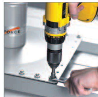
standing seam roof system installation
