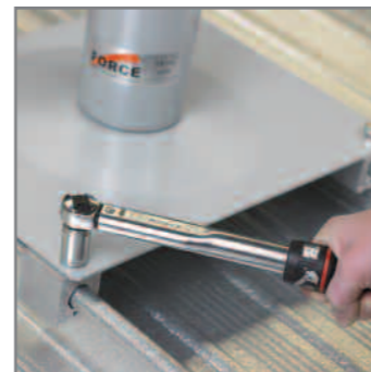
standing seam roof system installation
