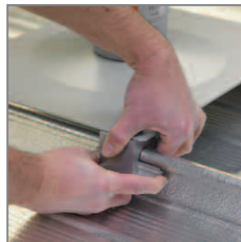
standing seam roof system installation
